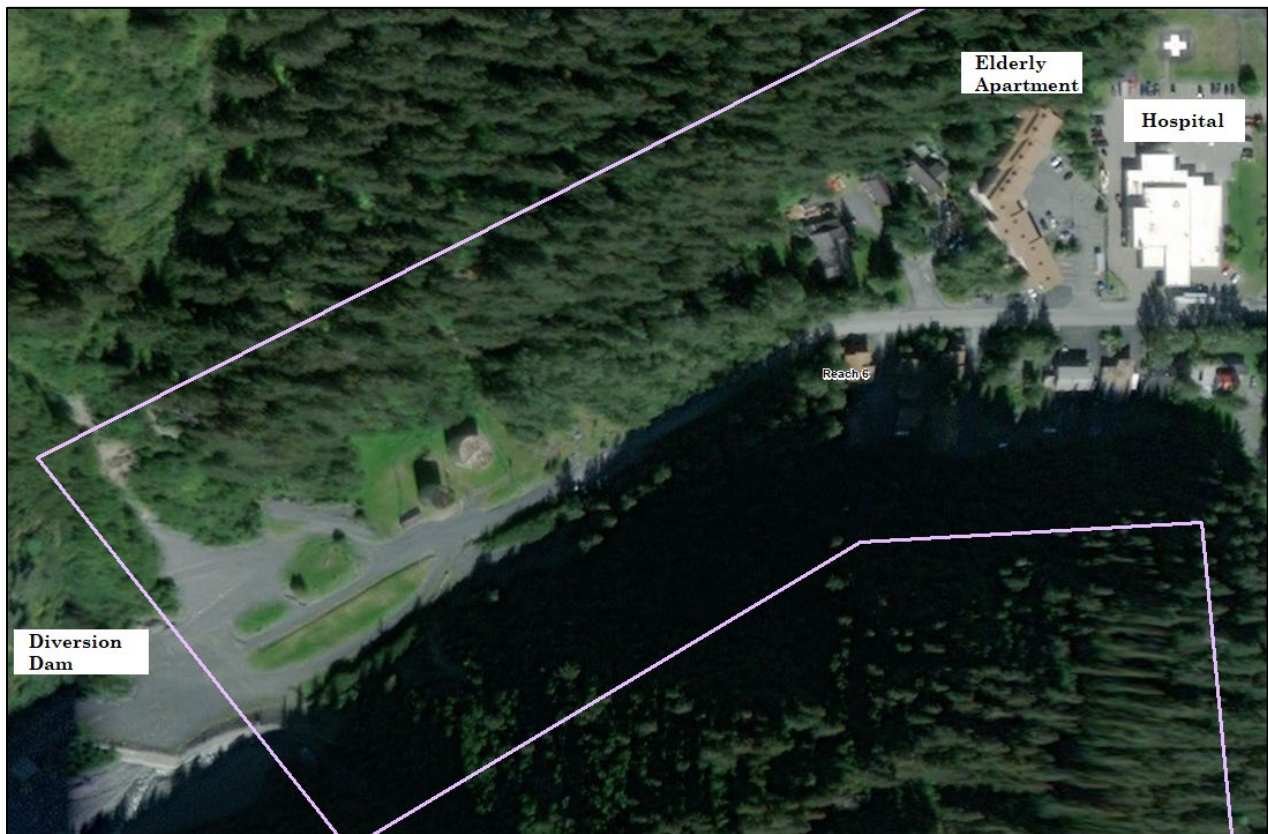
Figure 3. Seward Critical Infrastructure
